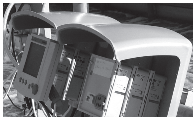
IQ SENSOR NET under sun shield SSH/IQ
